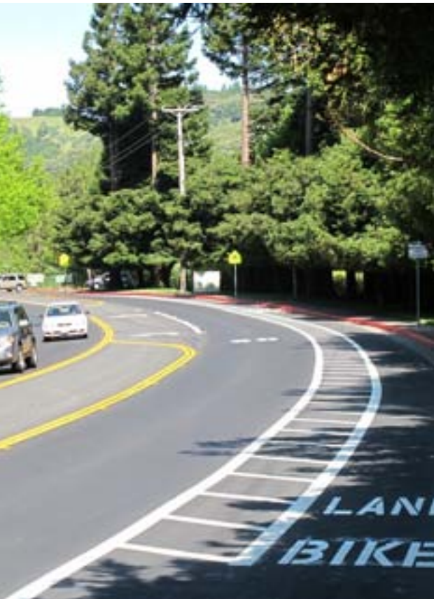
Example of a road diet. Road diets have been successful in changing fast, auto-oriented roadways into multimodal corridors.
