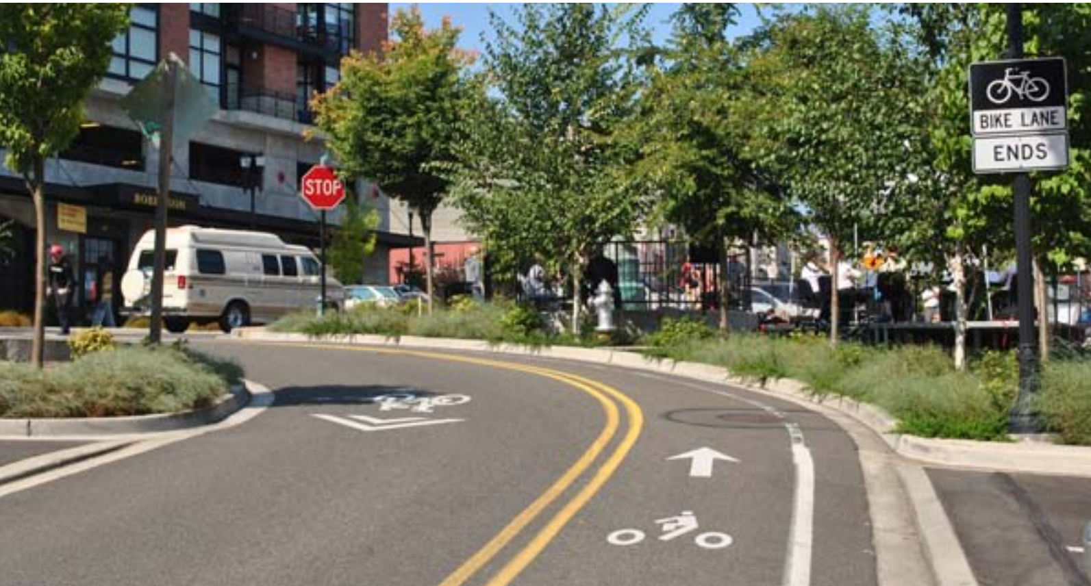
Being creative with funding sources can be the difference between implementing bicycle facilities and having gaps in the network. This contraflow bike lane paired with a sharrow completes a key connection in Tacoma, WA.
