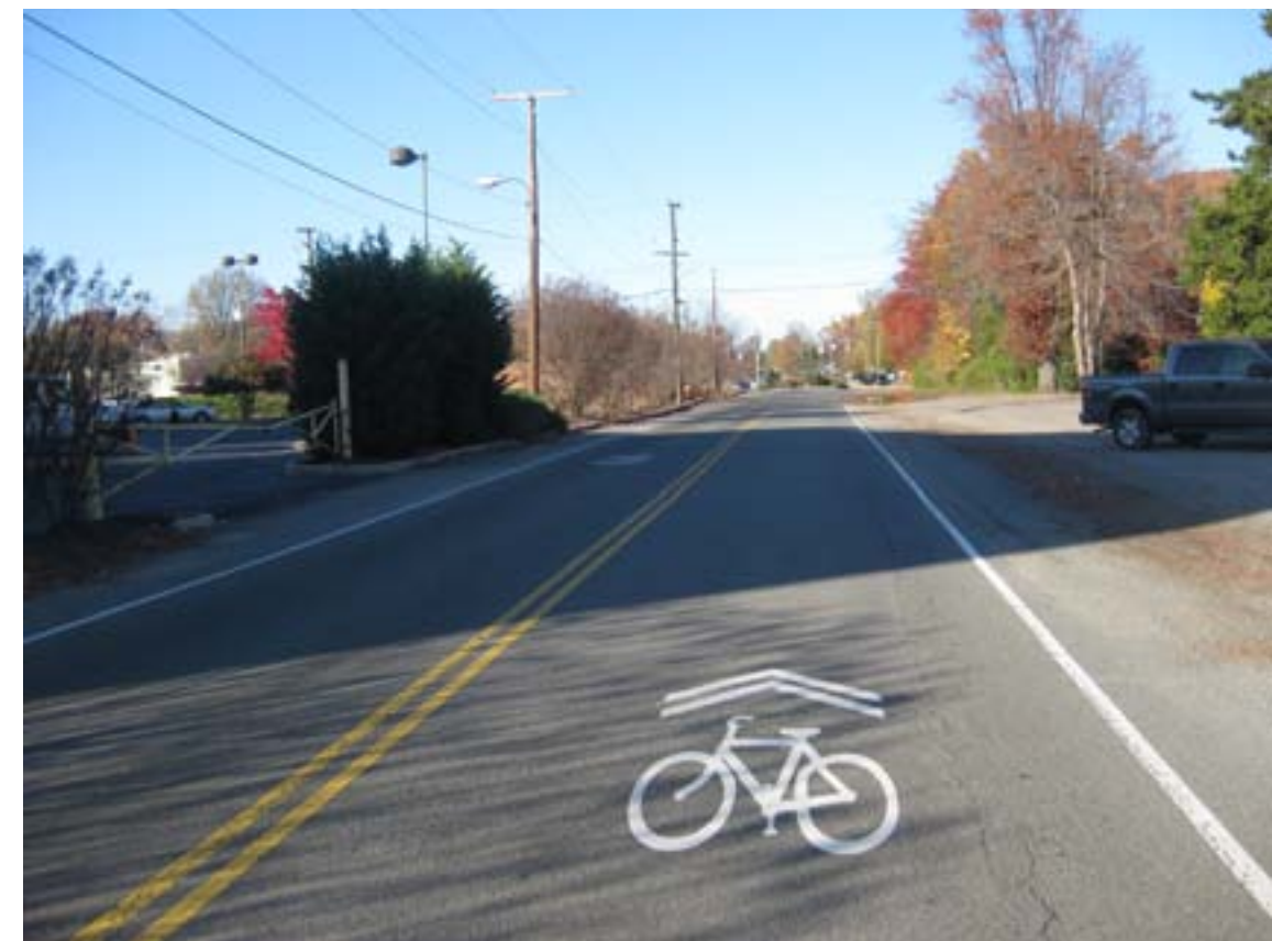
Hermitage Road is an example of an existing facility marked with sharrows.
