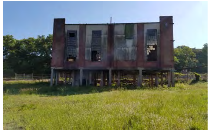
View of Building #2
