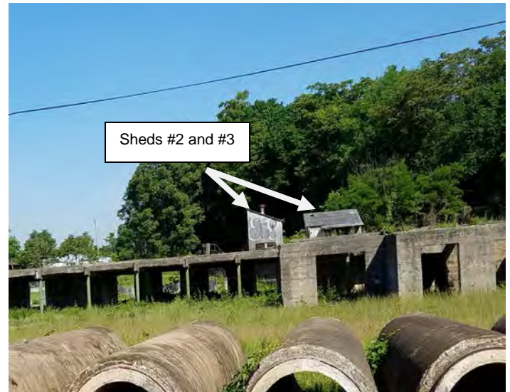
View of Shed # 2 and Shed #3
