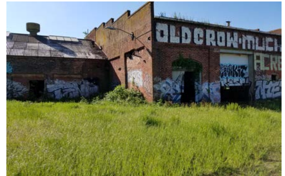
View of Building #1
