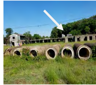
View of Sheds #2 and #3
