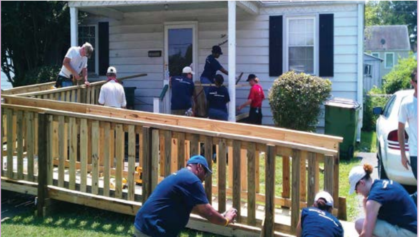
Project: HOMES - adding a ramp to allow residents to age in place.
