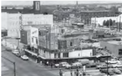
Construction of Covention Center
