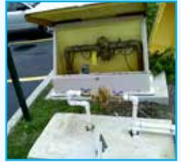
Placed just downstream of a water meter to an establishment, they can protect the public water system from any contamination that may occur within the entire establishment's plumbing system.
