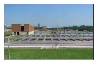
**DESCRIPTION & SCOPE:** This project provides for the upgrading of equipment and process control systems at the Wastewater Treatment Plant. The wastewater system serves approximately 58,000 customers in the City, Henrico, northern Chesterfield and Goochland counties.
