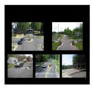
**DESCRIPTION & SCOPE:** This project provides for the installation of traffic calming devices including residential circles, chokers, speed cushions, splitters and raised crosswalks.
