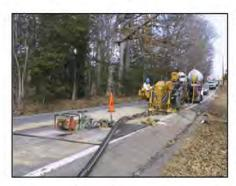
**DESCRIPTION & SCOPE:** This project provides for the replacement of gas mains, services, meters, and regulators. The primary projects included in this program are replacement of old gas mains, replacement or renewal of old gas services and response to water infiltration. Also included are projects to renew or replace mains in conjunction with projects being done by other City agencies or the State. It is estimated to replace 120,000 feet of main and 2,100 services in FY 2014.
