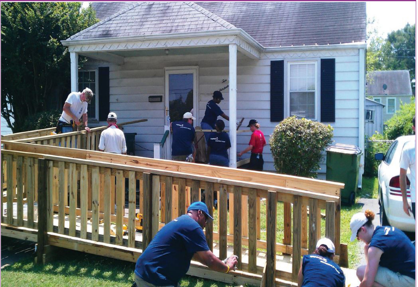
Project: HOMES - adding a ramp to allow residents to age in place.
