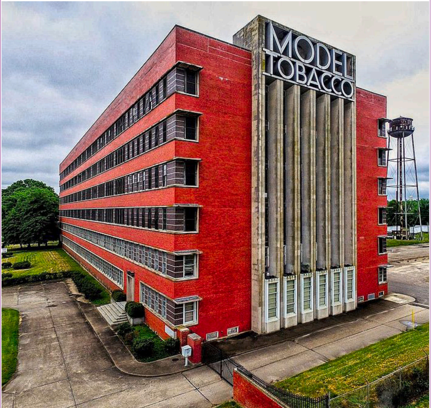
The Model Tobacco Building in Manchester to be rehabilitated into affordable housing.
