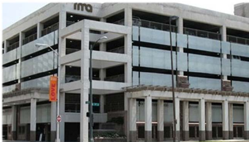
Expressway Parking Deck
