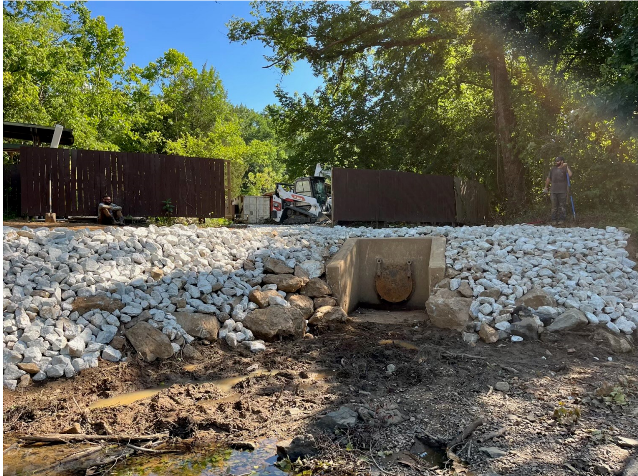
Figure 3-1: Restabilized CSO 17 Outfall
