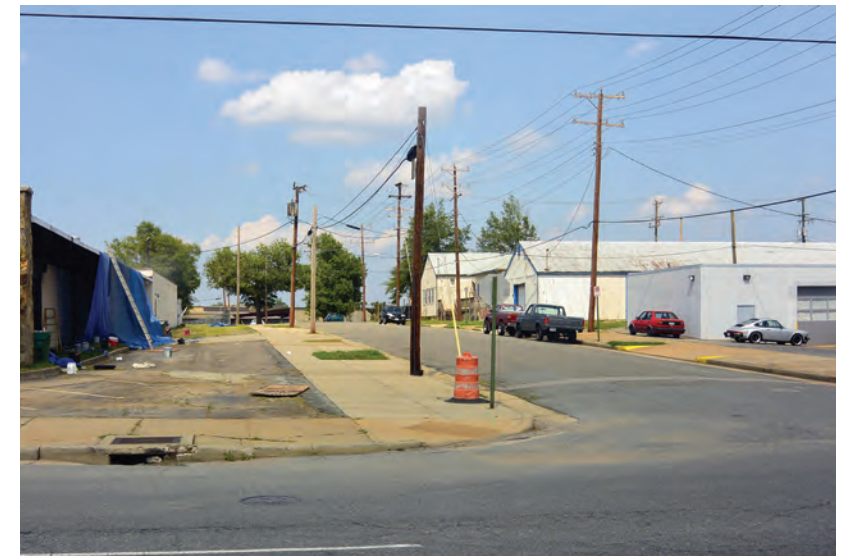
EXISTING CONDITIONS OF THE INDUSTRIAL AREA ALONG BROOK ROAD
