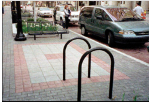
Figure 14: U-racks Installed on a Sidewalk (Photo from Cycle Safe (tm) Bike Racks)
