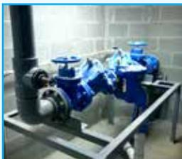
distribution system supplying it. Back-pressure can result from an increase in pressure on the customer's side—due to pumps, steam boilers, or other means—or from a decrease in pressure in the city's distribution system due to water line flushing, fire fighting, or water main breaks.
