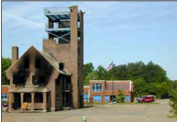
**DESCRIPTION & SCOPE:** This project funds the stabilization and repair of the Richmond Fire Department Burn Tower, which has been closed by the City Inspector until repairs are completed. The structure is used in the training of firefighters and is mission critical.
