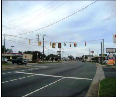
**DESCRIPTION & SCOPE:** This project provides improvements to existing traffic signals by upgrading aged and damaged equipment. Improvements range from converting span wire designs to mast arms for improved visibility and maintenance to installing new vehicle detectors for improved operations (such as fewer unnecessary stops and less delay and vehicle emissions).
