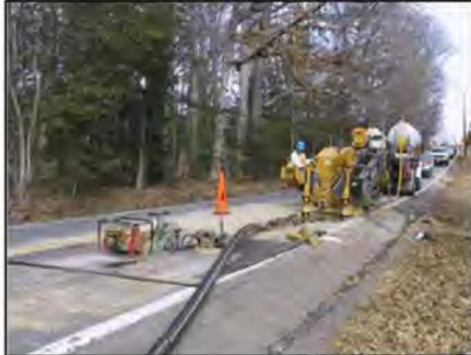
**DESCRIPTION & SCOPE:** This project provides for the replacement of gas mains, services, meters, and regulators. The primary projects included in this program are replacement of old gas mains, replacement or renewal of old gas services and response to water infiltration. Also included are projects to renew or replace mains in conjunction with projects being done by other City agencies or the State. It is estimated to replace 120,000 feet of main and 2,100 services in FY 2014.
