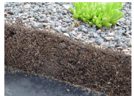
Example of a vegetated "green" roof cross section source: B. Hunt, NCSU
