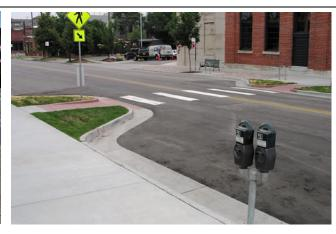
One of the ways to improve pedestrian crossings is to reduce the distance the pedestrian has to travel through the installation of curb bump outs like the ones shown in *Figure 11* above. These structures provide a visual cue to motorists to slow down by constricting the roadway visually and lessen the distance a pedestrian has to cover to clear the roadway.
