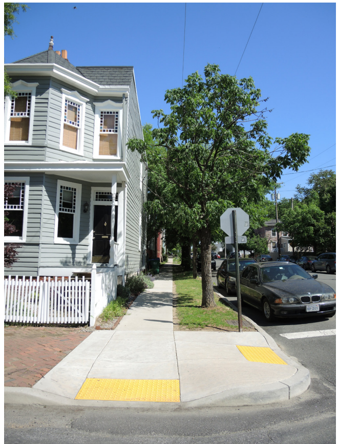
A new sidewalk in Church Hill includes ADA-compliant ramps at the intersection.
