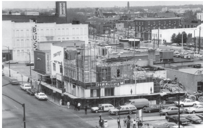
Construction of Convention Center
