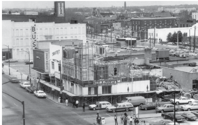
Construction of Covention Center
