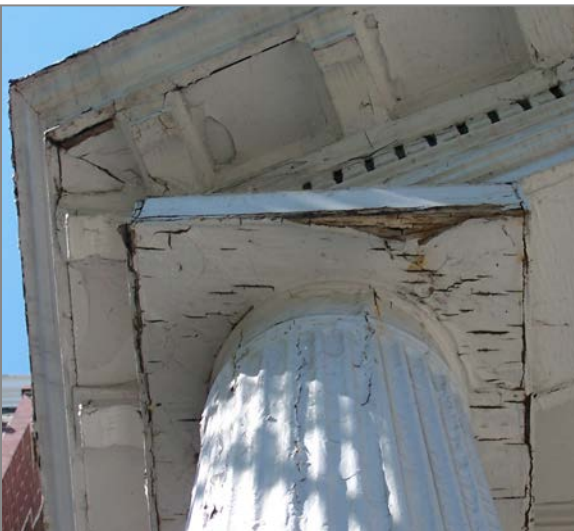
Cracked, peeling or blistered paint signals excessive moisture, improperly prepared paint surfaces or chemical incompatibility of paint layers.
