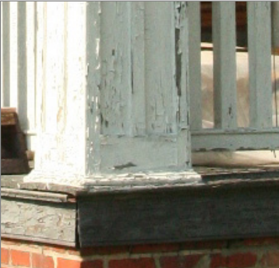
Cracked or warped boards can result from long-term exposure to the extremes of weather or from pressure stresses.
