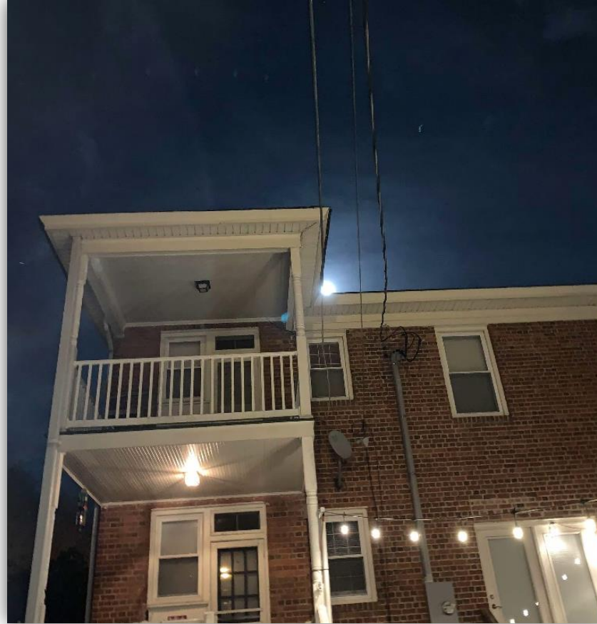
Rear Picture Location of Meter
