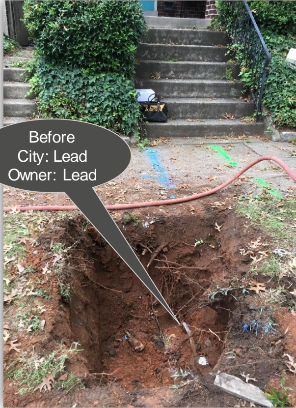
Excavation of Water Service – Ex. Lead
