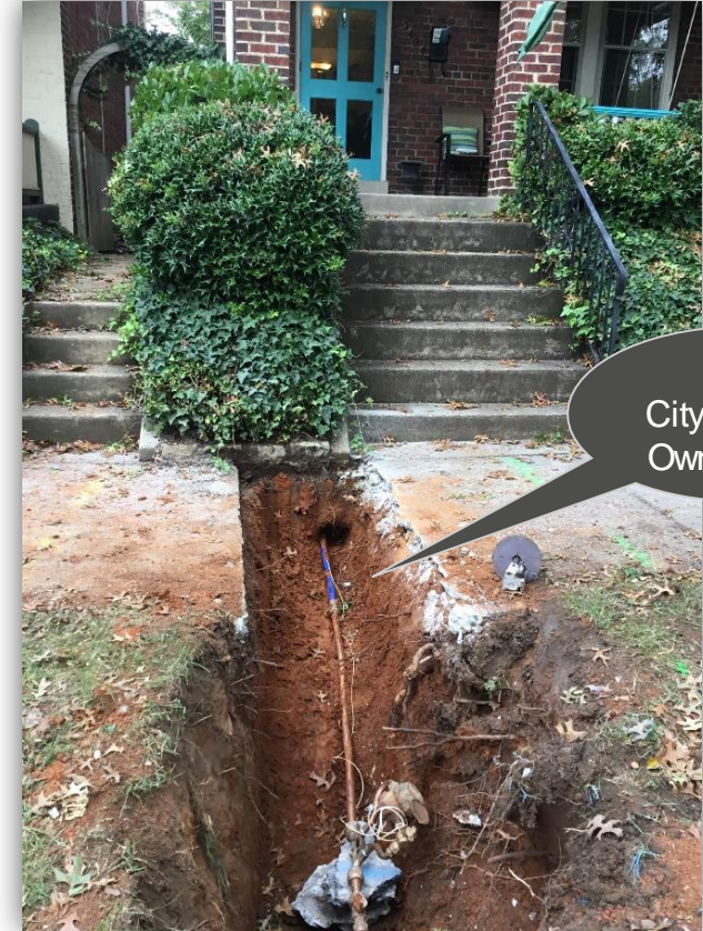
Excavation of Water Service – Replaced
