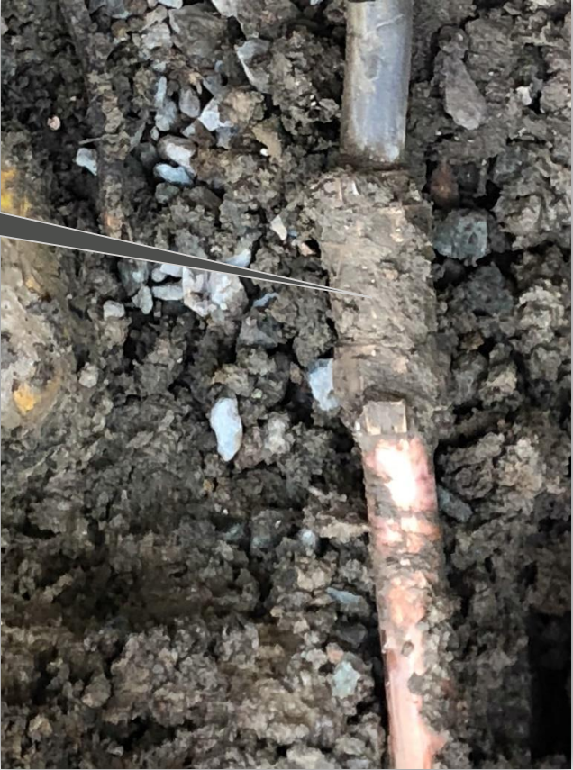
Closeup of Lead Service
