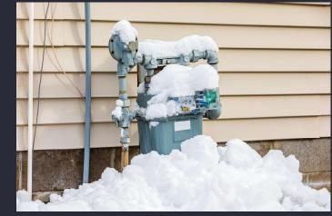
• DO remove excessive snow, ice, dirt and mulch from your meter. • DO have at least a 3 foot clearance around your gas meter to allow the utility provider easy access.
