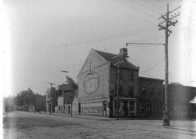
SW Corner of N. 18th and E. Broad Streets, ca. 1911 Valentine Museum
