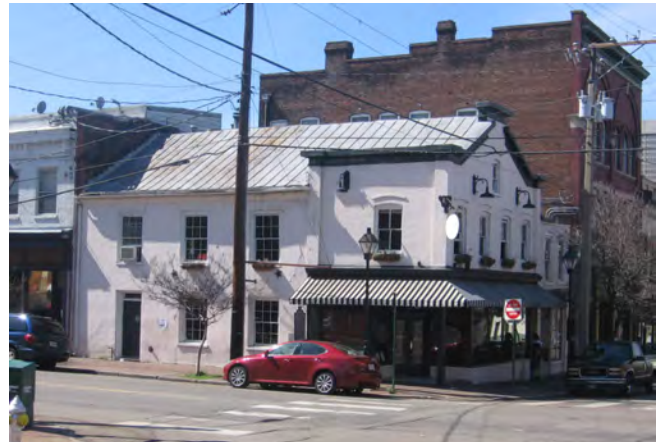
Whitlock’s Factory, built ca. 1817 1719 E. Franklin Street
