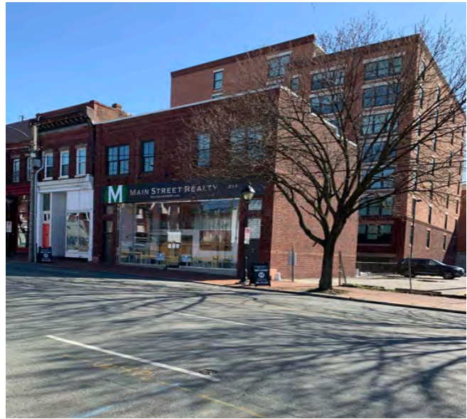
1817 E. Main Street and 12 S. 19th Street, constructed in 2016
