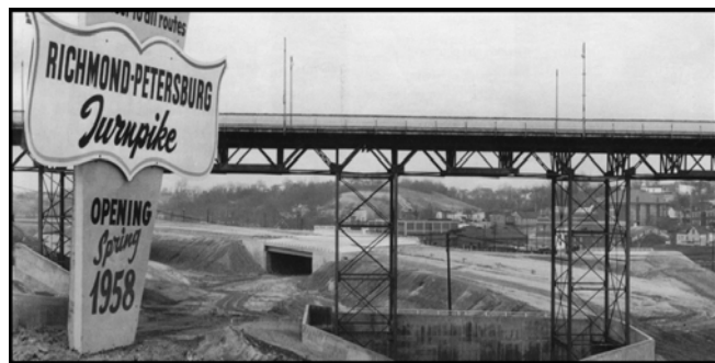
Richmond-Petersburg Turnpike under construction, ca. 1957; Marshall Street Viaduct in the background Valentine Museum
