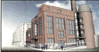
Lucky Strike Apartment Building
