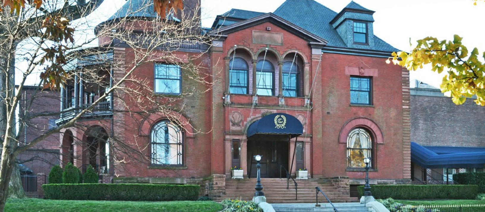
Commonwealth Club Historic District. Calder Loth, 2020
