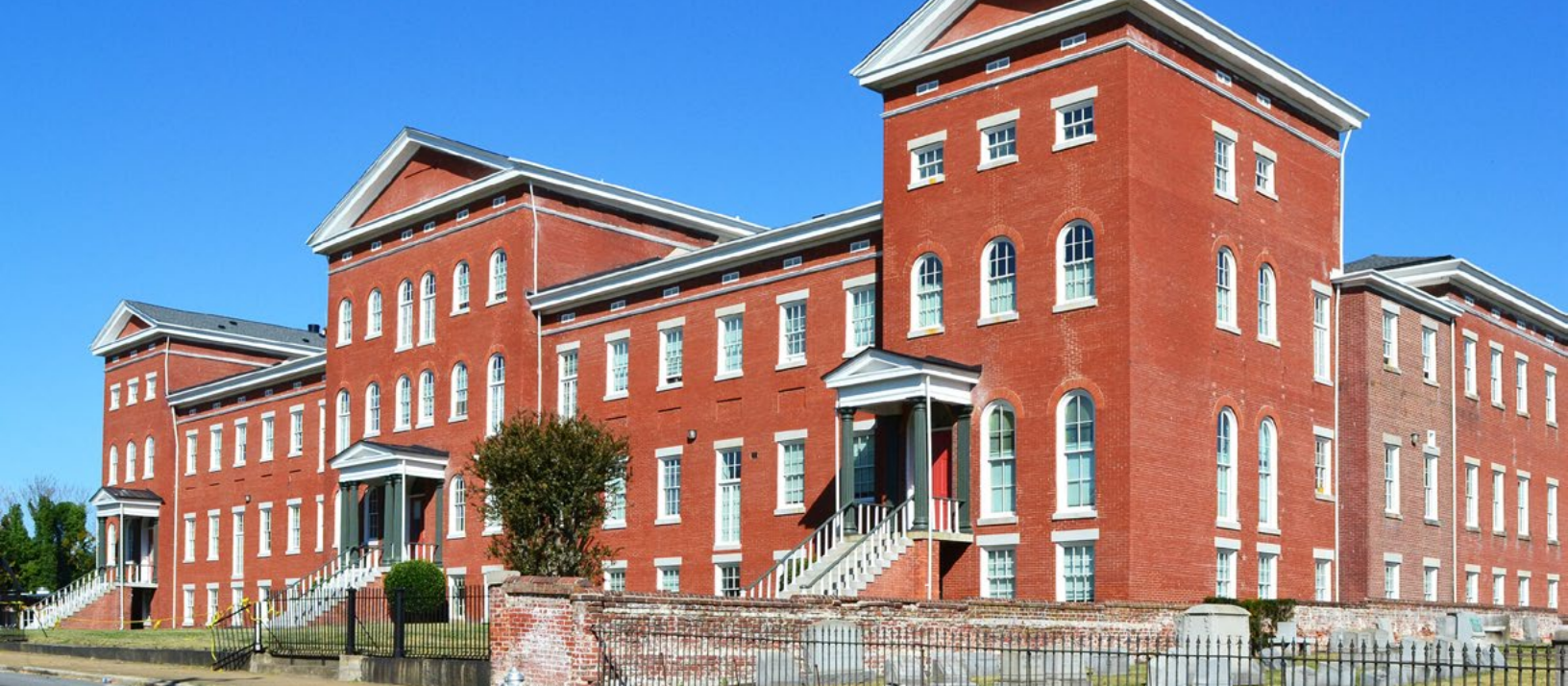
The Almshouse. Calder Loth, 2023
