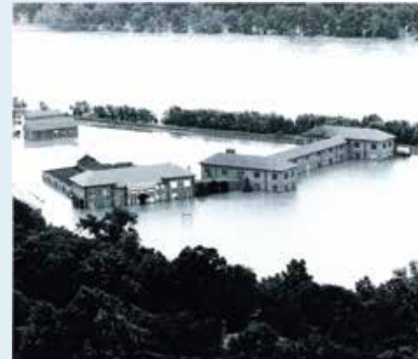
Richmond's Water Treatment Plant during Hurricane Agnes in 1972
