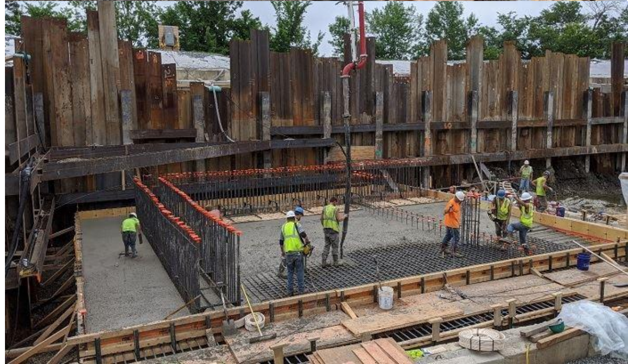
Photos of Davis Brook CSO Storage Tank | Bangor, ME
