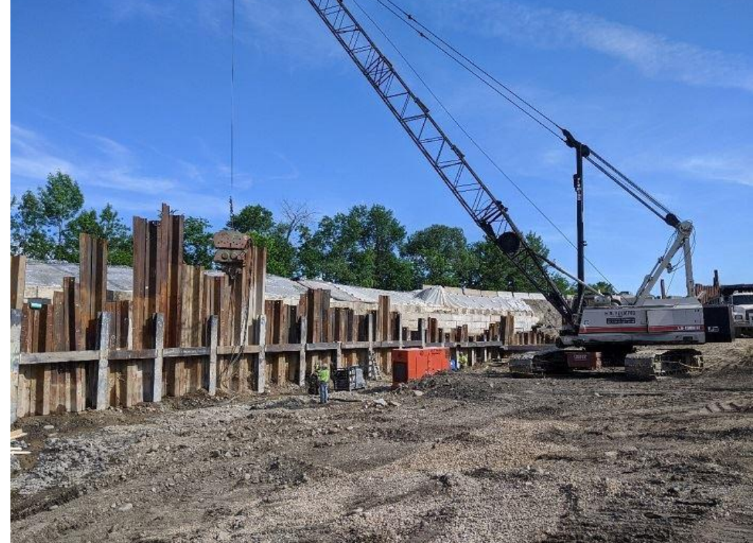
Photos of Davis Brook CSO Storage Tank | Bangor, ME
