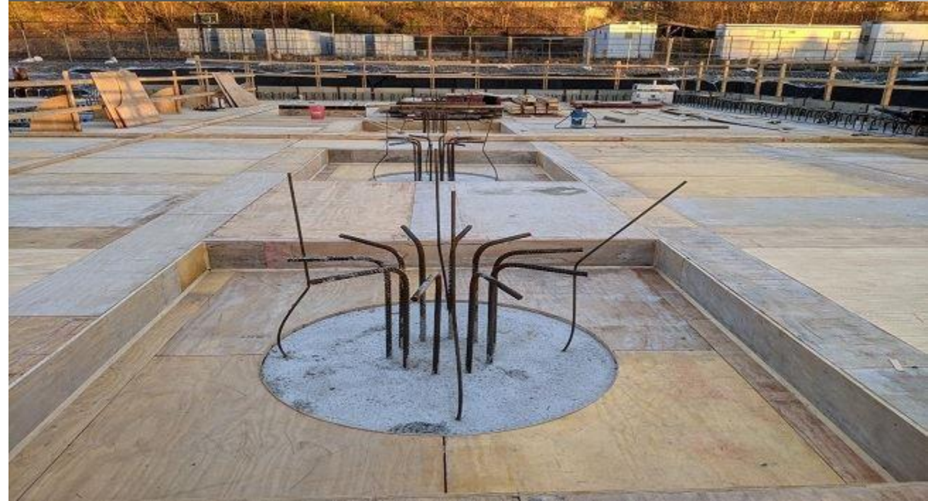
Photos of Davis Brook CSO Storage Tank | Bangor, ME
