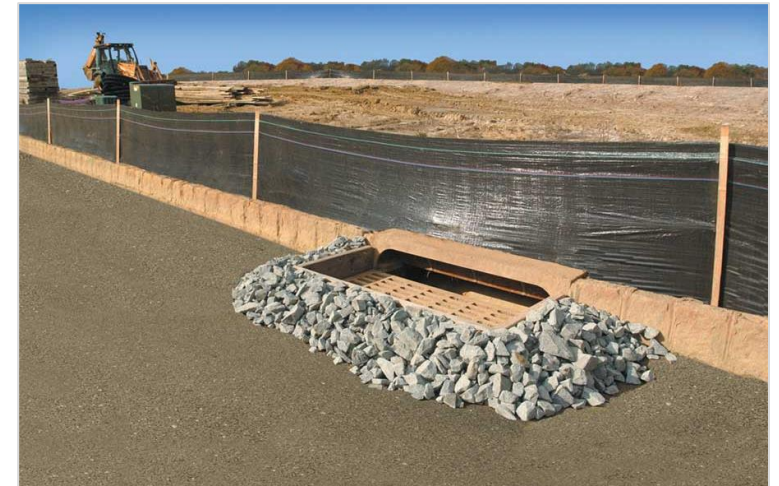
Erosion & Sediment Control
