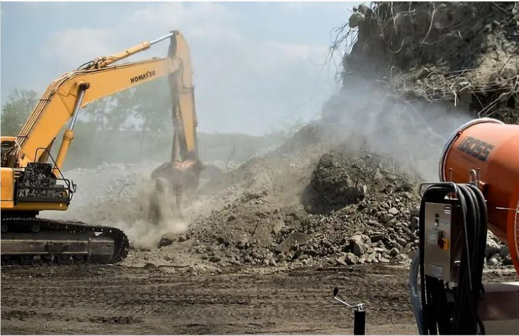
Excavate Soil in Saturated Conditions
