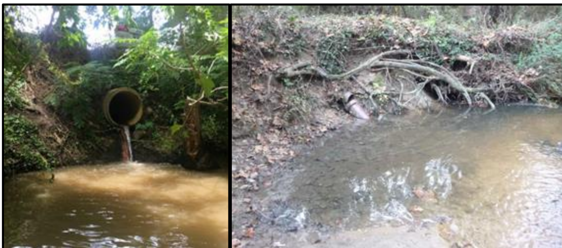
Figure 4-7. Pre-restoration images of Little Westham Creek.
