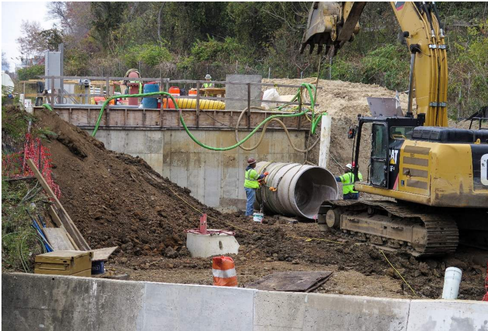
Construction of Outfall 004 Regulator and overflow pipe (Interim Plan project) Fall 2025
