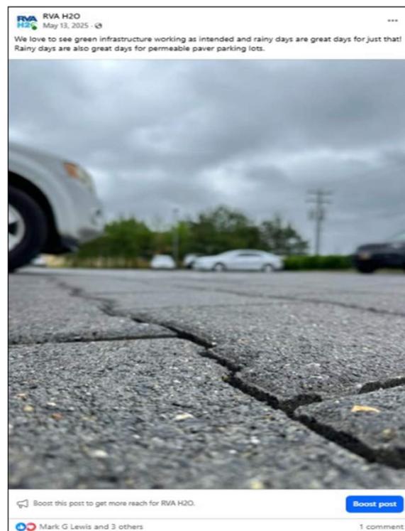
Figure 3-7: Permeable Pavement Post on Facebook on 5/13/2025
