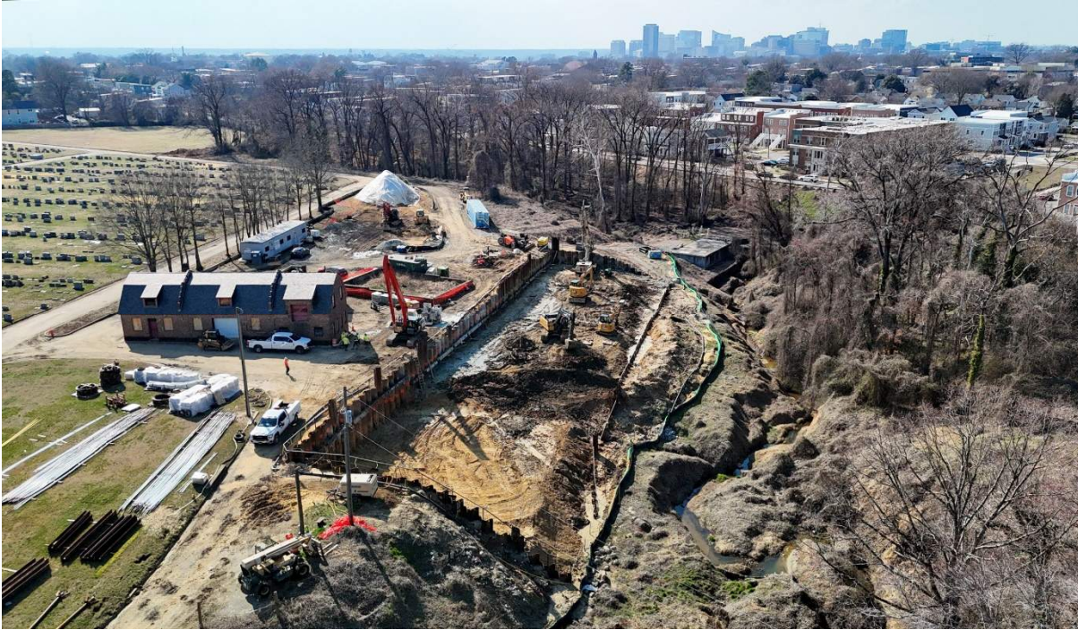
Construction of CSO 31 storage tank (Final Plan project) Winter 2025
