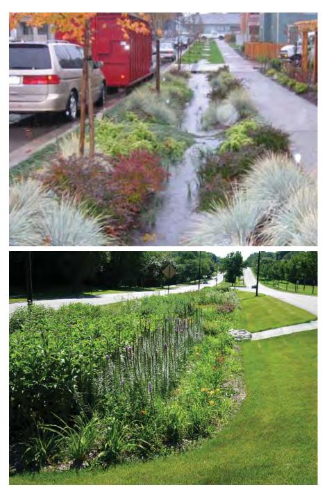
Figure 8.8: Bioswales alongside the road and in the median
