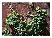
while picturesque, climbing vines can prematurely weaken a brick wall by aiding in the deterioration of mortar joints.
