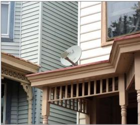
Satellite equipment should not be located at the front of a building.
